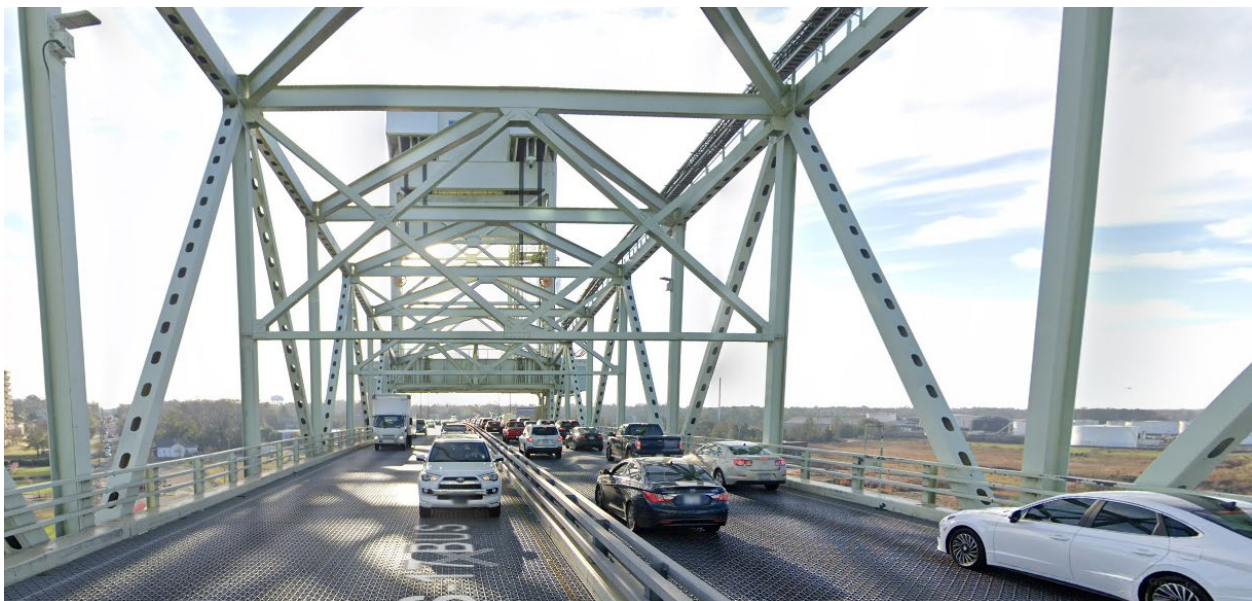
Figure 1: Existing Conditions on the Cape Fear Memorial Bridge
